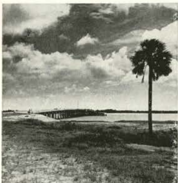
One of five modern bridges on the route
