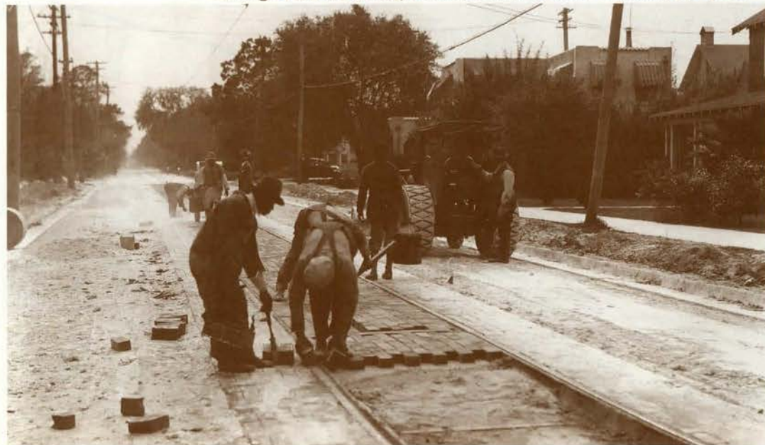
Paving Herschel Street, between Seminole and Avondale, ca. 1926
