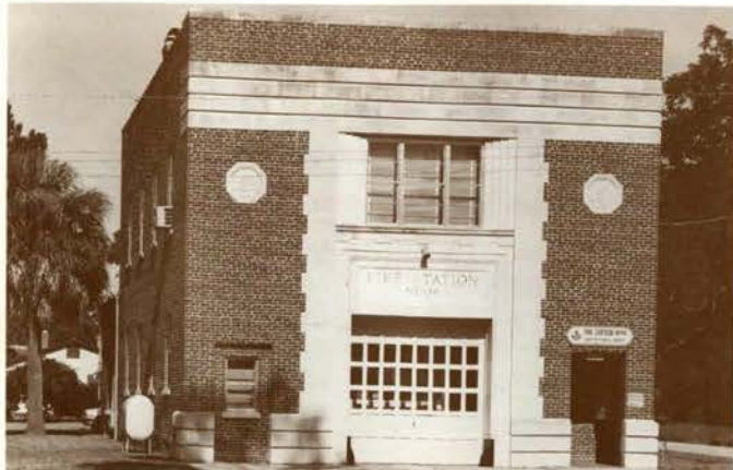
Fire Station #14, 4242 Herschel St. (built 1933)
