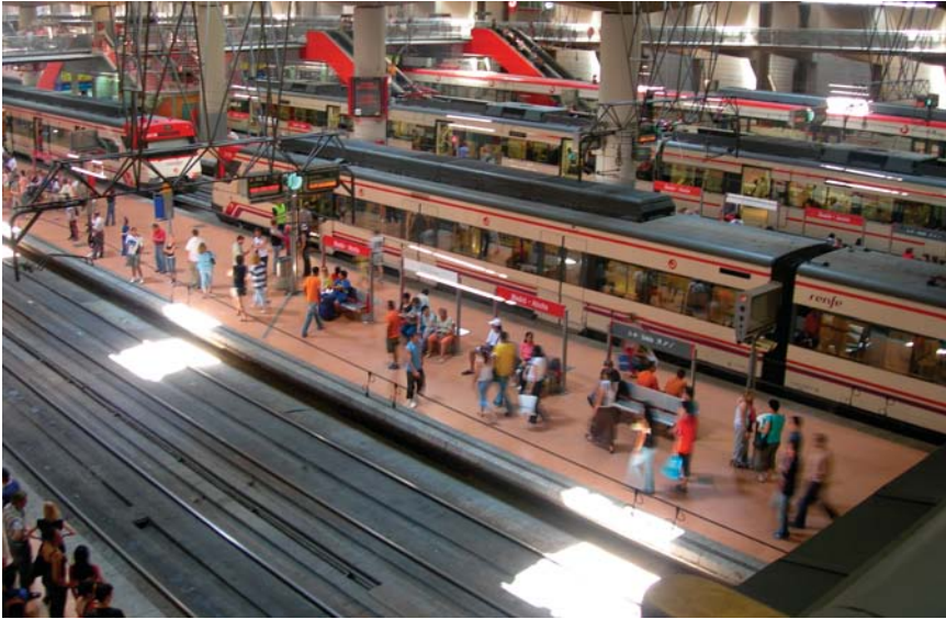
Figure 3. Atocha Station, Madrid, Spain. Photograph by Mike Chamberlain. Reprinted with permission from the artist.
