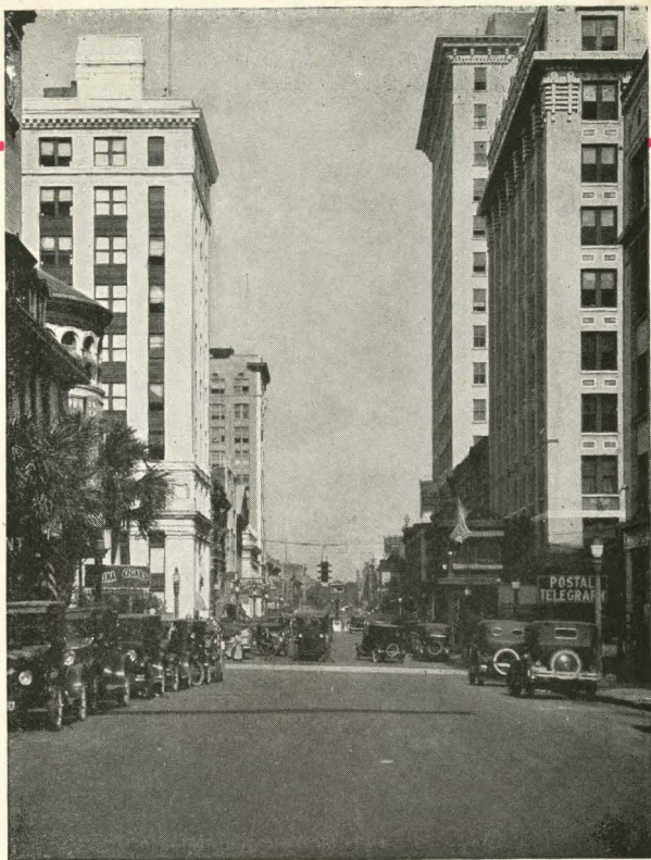
Looking East on Forsyth Street Jacksonville's Financial District
