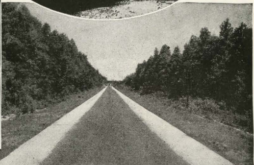
A typical road—concrete—good in all weather
