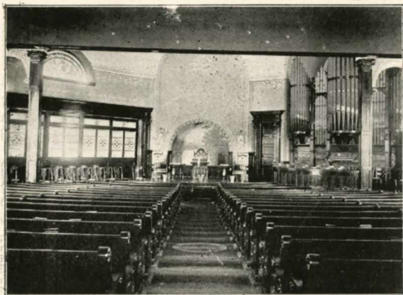
INTERIOR VIEW OF THE MAIN AUDITORIUM INTO WHICH THE SUNDAY SCHOOL AND LECTURE ROOM AT THE LEFT MAY BE OPENED
