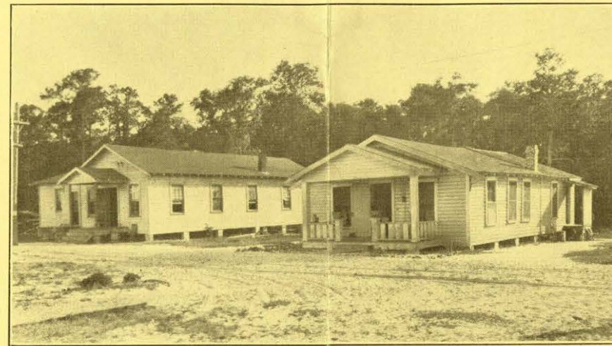
COTTAGES BUILT BY STUDENTS
