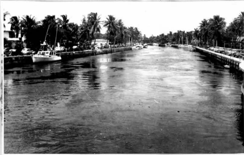
New River - looking east from Andrews Avenue bridge.
