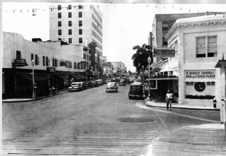
Andrews Avenue looking north from New River bridge. Ultimately, with completion of Third Avenue improvements and bridge this street should be "one-way" north to south.
