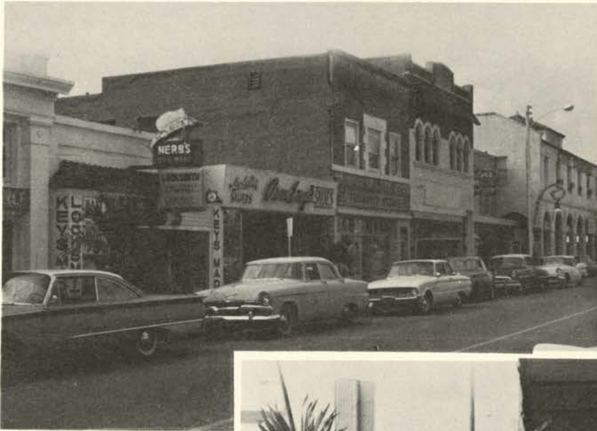
STORE FRONTS ON LAKE AVENUE NEEDING REHABILITATION
