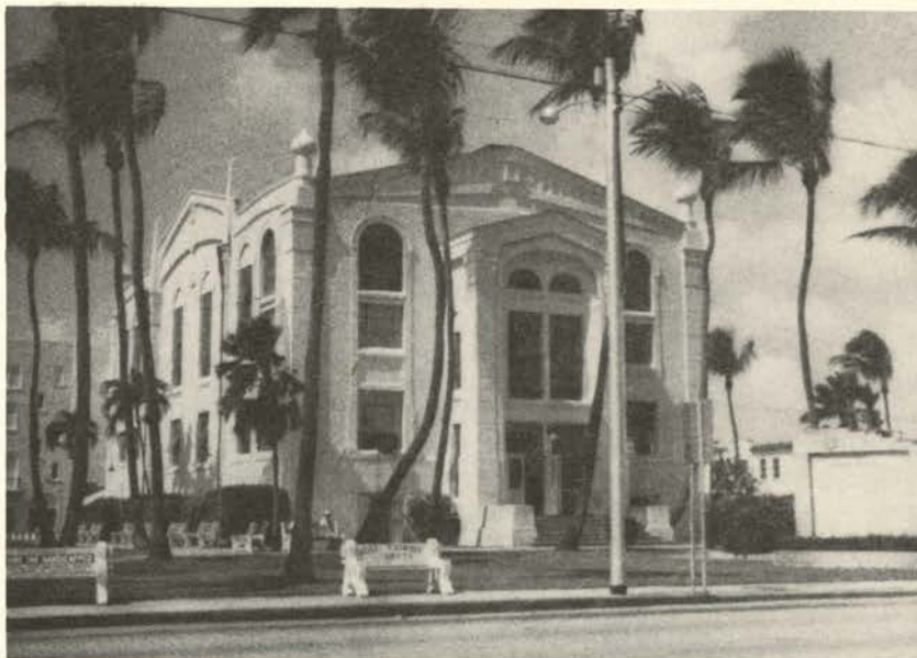
THIS STRUCTURE SHOULD BE REPLACED WITH ONE MORE MODERN AND SERVICEABLE
