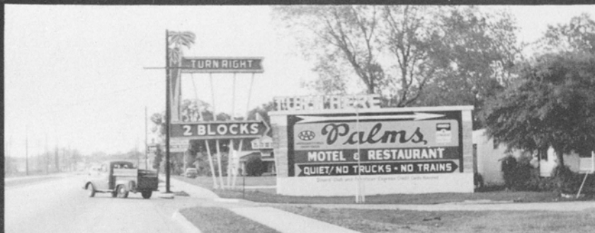
BILLBOARDS ENCROACHING ON RESIDENCE AREA
