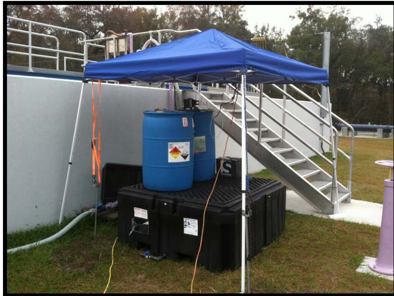
Figure 32 - PAA Barrels on Containment System
