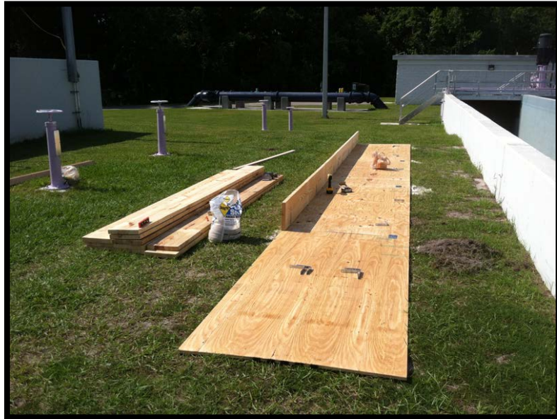
Figure 36 - Leveling and Construction of Model CCC
