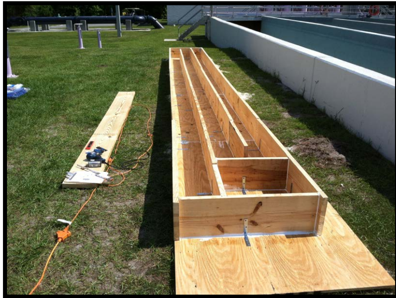
Figure 37 - Completed Framework of Model CCC
