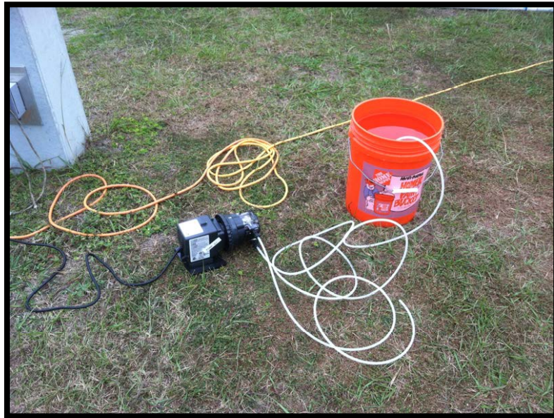
Figure 43 - Chemical Dosing Pump Calibration
