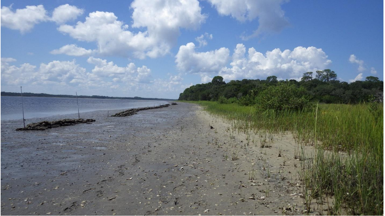
Figure I-2 Installed artificial reef segments along Wright's Landing Wright's Landing in the northern Guana Tolomato Matanzas National Estuarine Research Reserve. Photo was taken September 4, 2013 following the installation of the final segments on the southern end.
