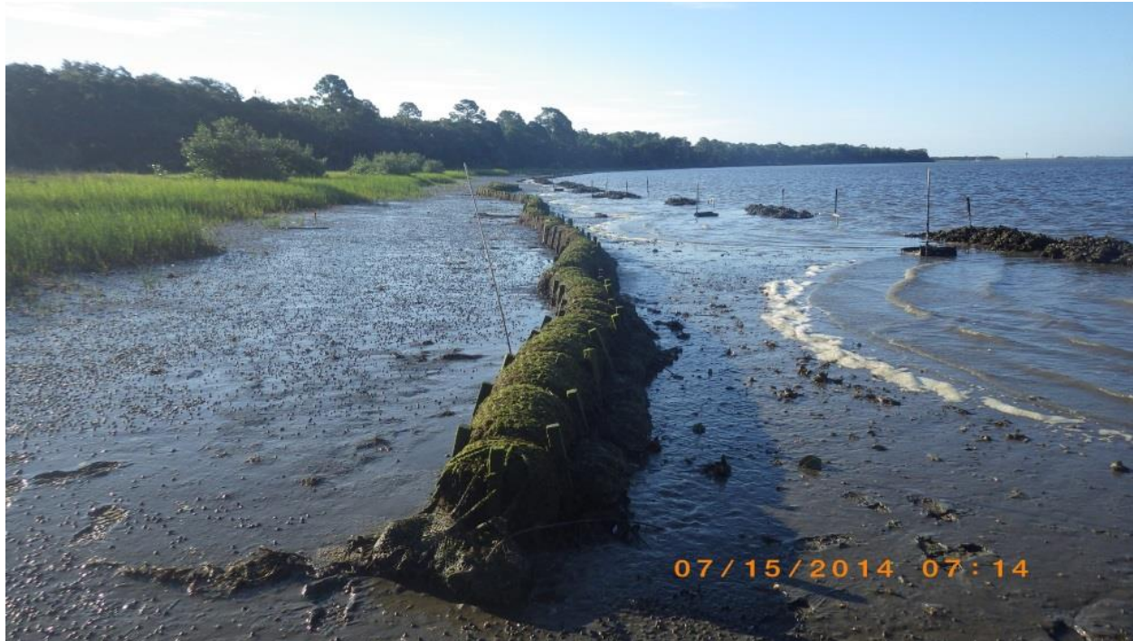
Figure 1-2 Deployed fiber (coir) logs along Wright's Landing in the northern Guana Tolomato Matanzas National Estuarine Research Reserve (30.0225250°N, 81.3262806°W) Florida, U.S.A. These logs were installed approximately 5 m from the existing Spartina marsh edge in the high intertidal zone. Logs were placed in 20-m arcs both behind constructed oyster reefs (pictured), and alone, along eroding shoreline.
