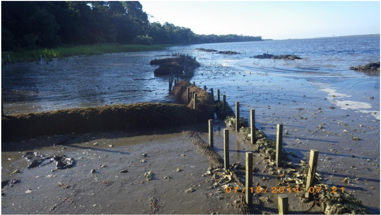
Figure I-5 Fiber log movement on the southern installation of the combination of artificial oyster reef and fiber log site along Wright's Landing in the northern Guana Tolomato Matanzas National Estuarine Research Reserve. Photo was taken July 15, 2014 after the installation of the fiber log only treatment was installed 100-m north of the artificial oyster reef.
