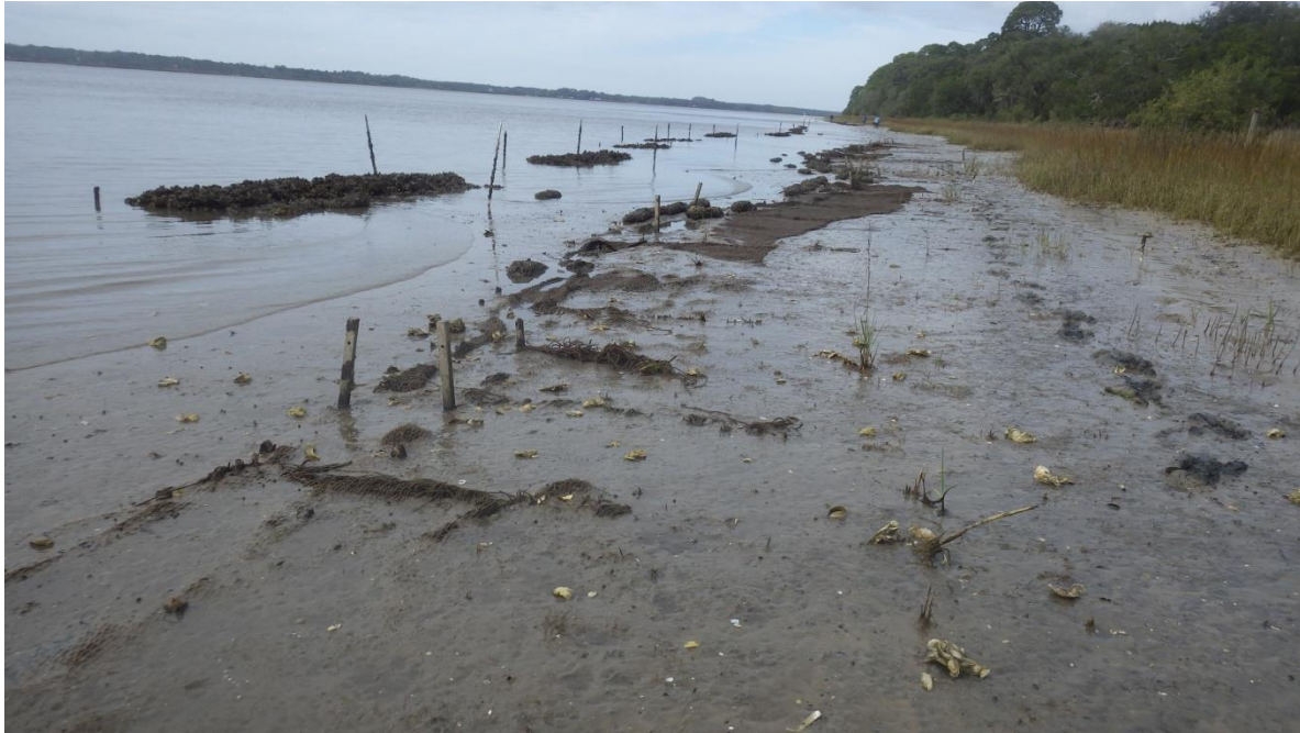
Figure I-8 After the partial removal of degraded fiber log material off the northern end of the artificial oyster reef along Wright's Landing in the northern Guana Tolomato Matanzas National Estuarine Research Reserve. This was the northern combination living shoreline site with both the artificial reefs and fiber logs. Photo was taken in January 17, 2015.
