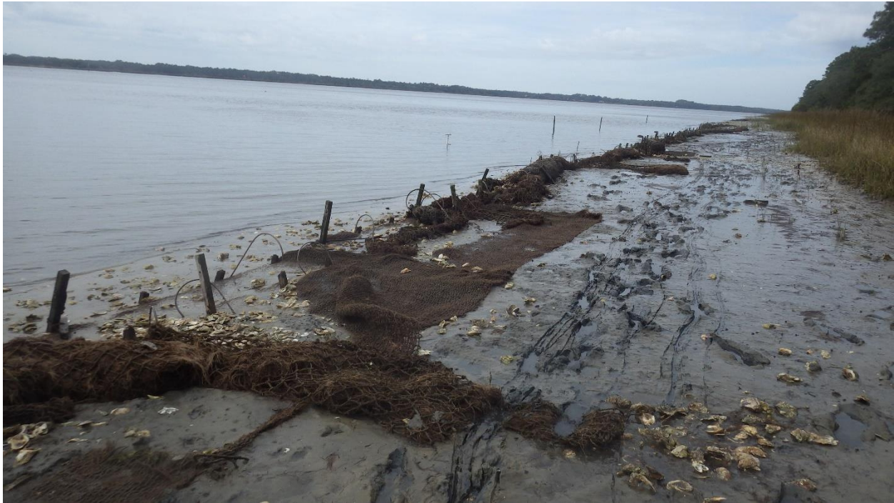
Figure I-7 Degradation and partial removal of the fiber logs installed 100-m north of the existing artificial oyster reef along Wright's Landing in the northern Guana Tolomato Matanzas National Estuarine Research Reserve. Photo was taken January 17, 2015. Logs were placed in 20-m arcs approximately five meters in front of Spartina marsh grass on unstructured eroding shoreline using wooden stakes and twine in July 2014.
